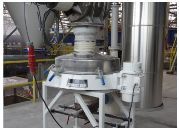
Figura 2. A 900mm diameter Russell Compact Sieve installed at Promat, Belgium to sieve a porous powder, Promaxon®-D.
