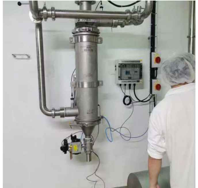
Figure 2. The installation of the Self-Cleaning Russell Eco Filter®
