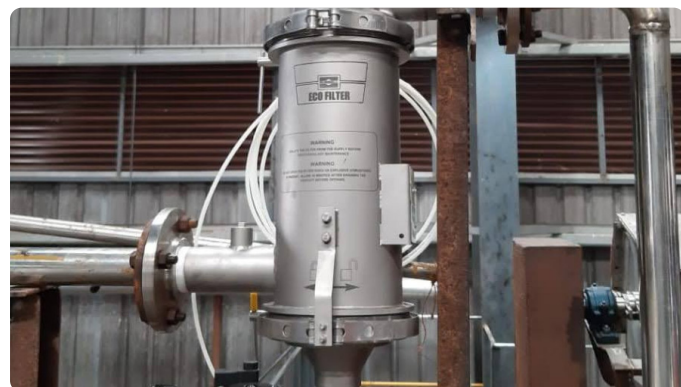
Installation of the Self-Cleaning Russell Eco Filter®
