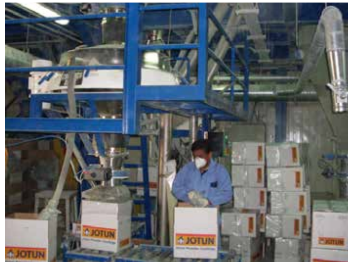
Figure 3: The Russell Compact Sieve® installed before the filling lines at Jotun UAE.
